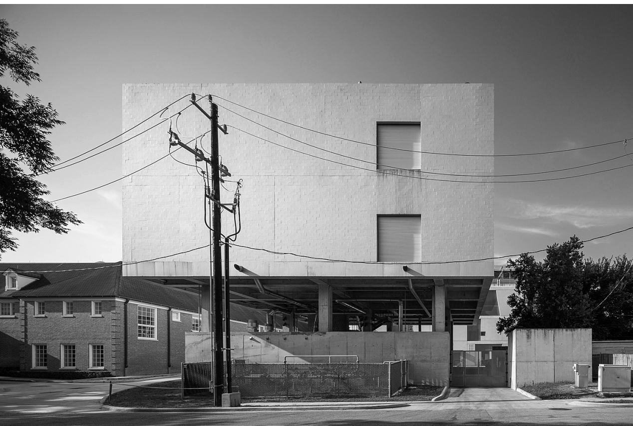
Steven Holl Architects, Museum of Fine Arts Houston Central Plant, Houston, Texas, 2020. Photo: Sean Fleming. Courtesy the architect.
